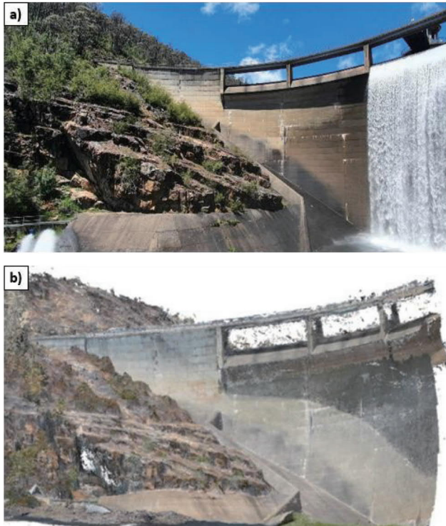
Fig. 2: Comparison of the outcrop on the right abutment a) as a photograph (November 2020); and b) as a screenshot of the point cloud generated from remote sensing (January 2020), presented in CloudCompare.
